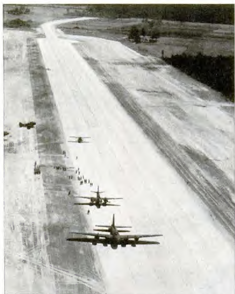
Planes land on runway made by widening highway with strips of paving
